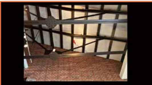
This building was located 4.6 km away from the epicenter. Though the shock wave bent the steel rafters supporting the roof inward, the building itself managed to survive.
